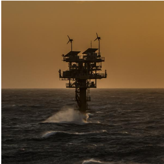
Figure 79: 3kW Wind turbines on an unmanned gas platform 53
