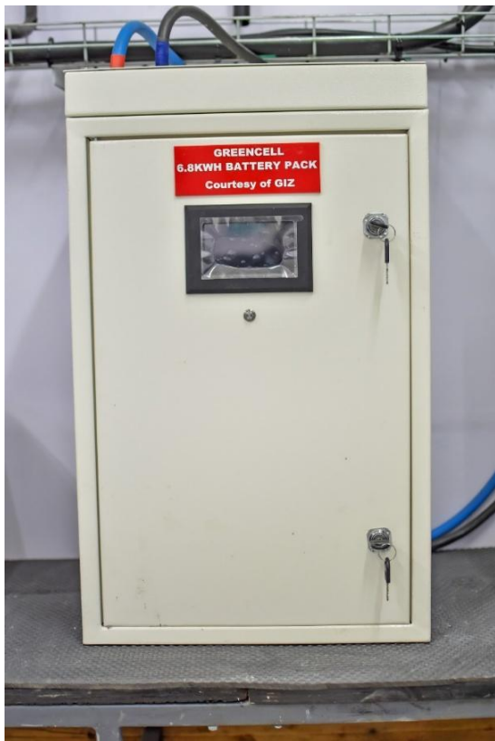
Figure 7 The 6.8 kWh GreenCell repurposed battery derived from a 2010 Nissan Leaf
