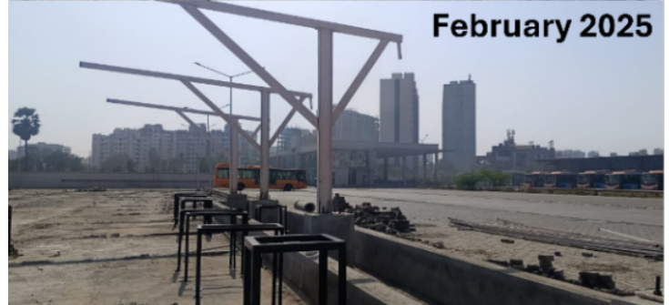
On going civil construction as of February 2025
