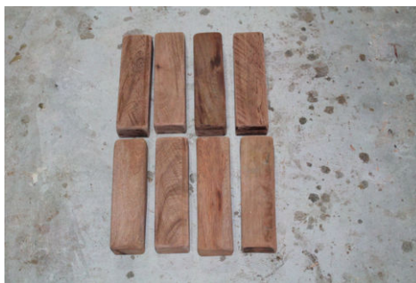
Figure 62: Eight hardwood blocks of the same size are cut as support for the cross-beams.
