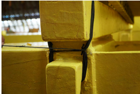
(d) Pull the wrap tight to further tighten the entire lashing. Finish off with overhand knots.
