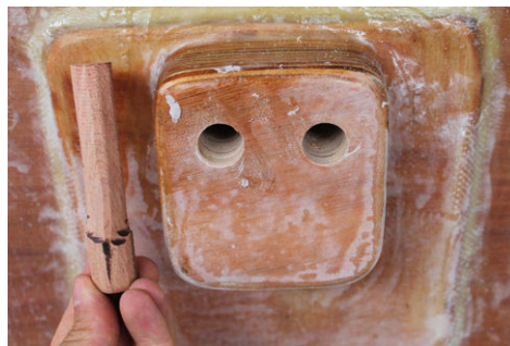
(c) Hardwood pins fit to the holes
