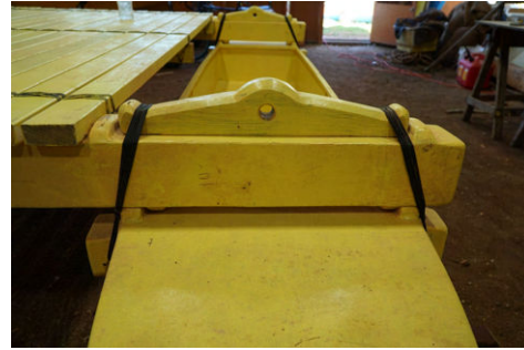
(b) Loop the lashing rope around the beam and beam cleat.
