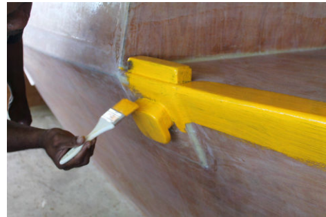
(b) Brushes are used for detail work only
