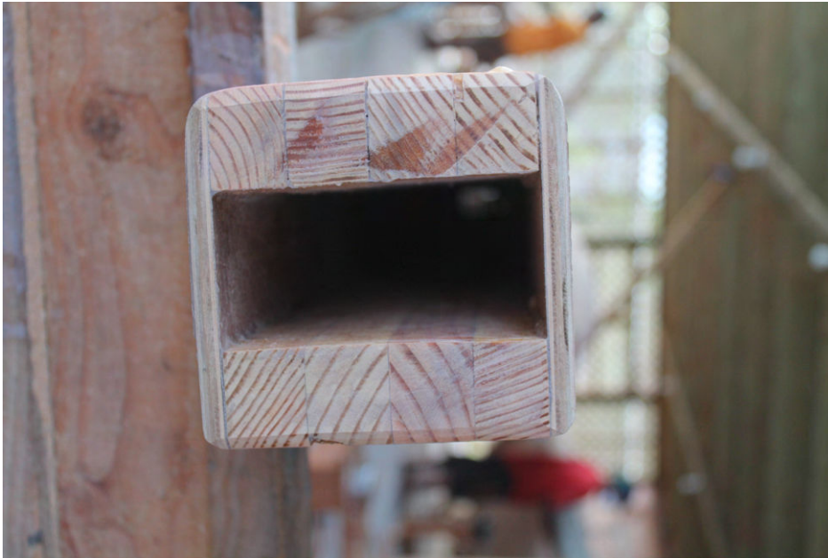
Figure 33: The rectangular and hollow cross section of the beams. The lumber is positioned on the top and bottom to take the bending loads while the vertical plywood works as a shear web.
