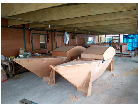
(c) The cabin sides are held in place by hot melt glue applied from outside. In the next step they will be fixed by fillets from inside permanently.
