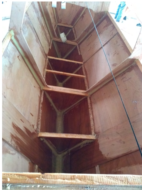
(c) The bunk-board support stringers are glued in using copper wire to temporarily fix them on the bent hull.
