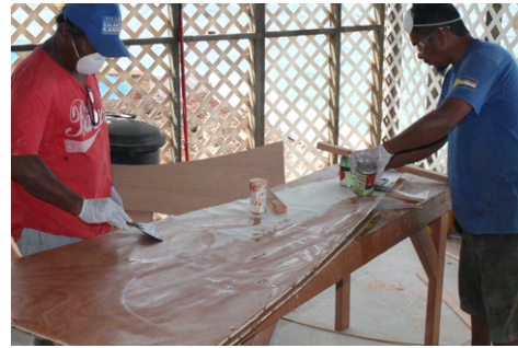
(b) The treatment is for reinforcement and for rot protection.
