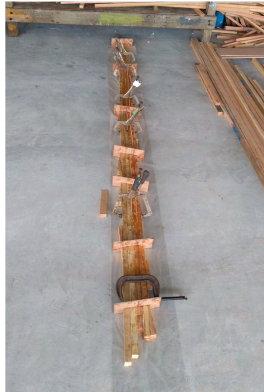
(b) Glue the lumber strips together to form a beam plank. Clamps keep everything in place.
