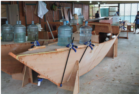
(a) The deck panels are glued on the shears and the bulkheads with thickened epoxy. Clamps and weights are used to temporarily hold them in place.
