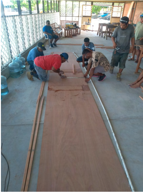
(a) Station lines are marked on the plywood.
