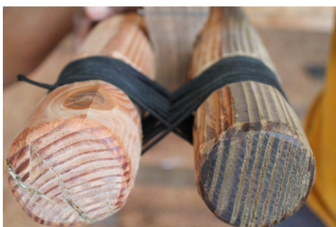
(c) Lashing finished and locked. To further tighten the lashing, the rope is now wrapped around the cross point of the figure-eight lashing.
