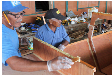
(b) Plenty of glue is spread on the bulkhead tops for a strong bond without any gaps. The glue is should squeeze out as an indicator of a good joint.
