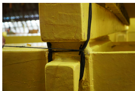
(d) Pull the wrap tight to further tighten the entire lashing. Finish it off with overhand knots.
