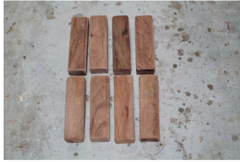
Figure 98: Eight hardwood blocks of the same size are cut as support for the cross-beams.
