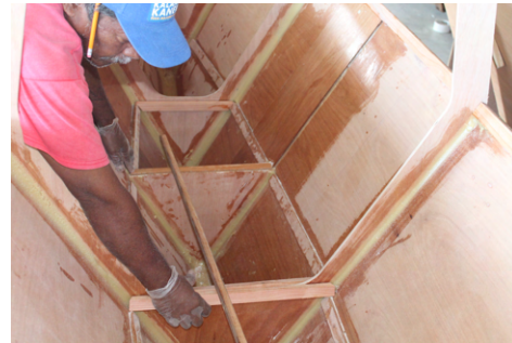
(b) Leveling the bunk-boards with a straight batten
