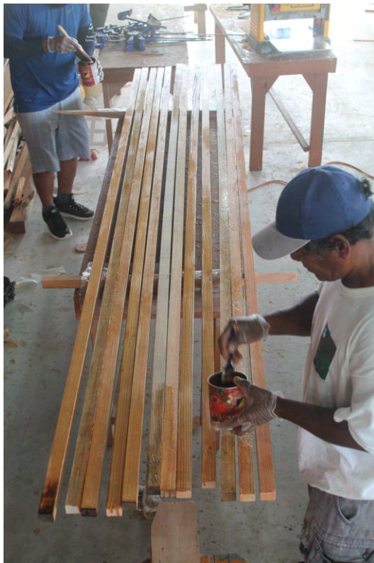
(a) Spreading epoxy glue on the lumber strips
