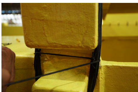
(c) Finish the lashing by wrapping the rope around the loops.
