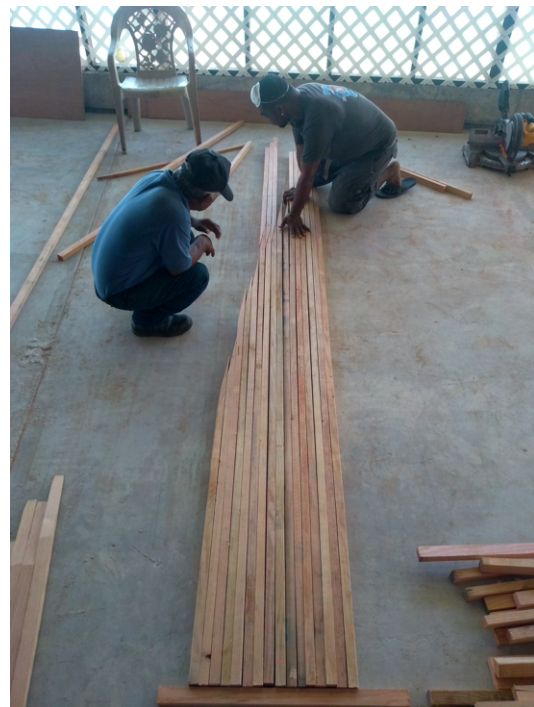
(c) Puzzling together full-length battens by using scarf connections.
