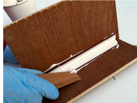
(d) A sharp spatula or wedge is used to clean off any excess epoxy mix.
