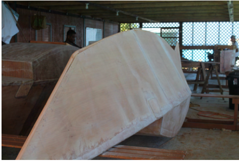
(a) Hull turned upside down and wires removed
