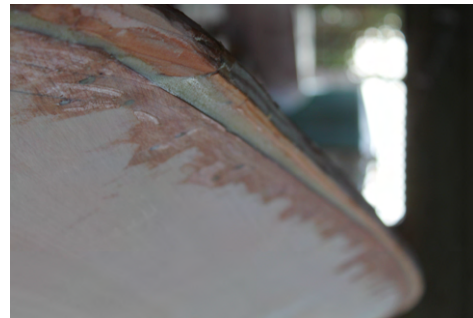
(d) All gaps in the transition from hull to keel are filled with thickened epoxy.
