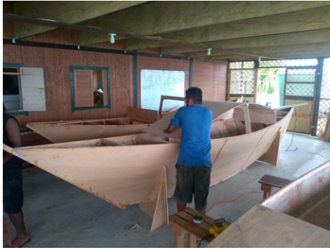
(a) The cabin roof is cut to the width of the bulkhead tops and placed at its desired position.
