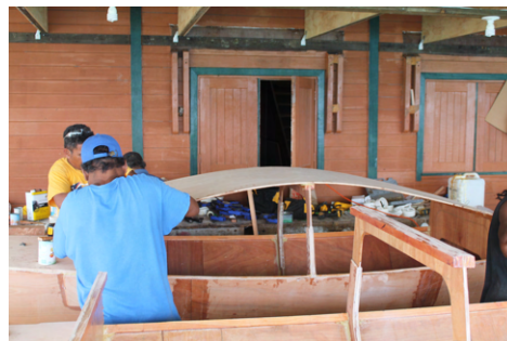
(d) The roof is bent down to its intended shape and fixed temporarily by clamps going around the bulkhead (not shown in the photo).
