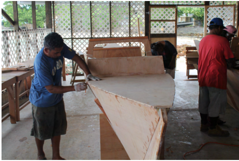
(a) The size of each deck panel is derived directly from the hull by placing it at the desired position and drawing a line around the outline.
