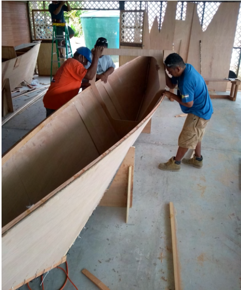
(c) The sheer is gently pulled apart to open the hull shell. The center bulkhead is carefully pushed inside. The sheer stringers should snap into the cut-outs of the bulkhead and lock in in place.
