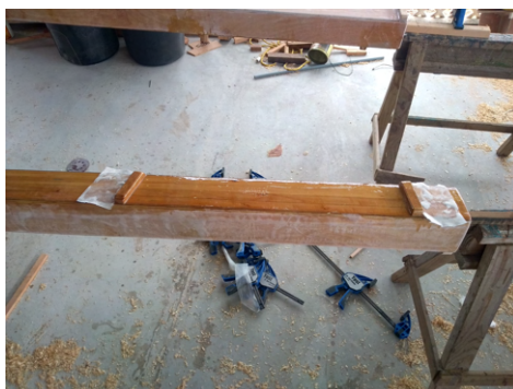
(c) Alignment blocks on the bottom of the beam: The contact area between the beam and hull is reinforced with additional glass.
