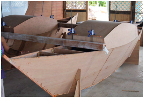
(c) Cabin sides and roof cut to the right dimensions and placed temporarily at the desired positions.
