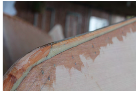
(e) All gaps in the transition from hull to keel and all holes from wires are filled with thickened epoxy.
