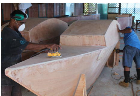
(d) The entire deck and cabin surface is sanded in preparation for glassing.
