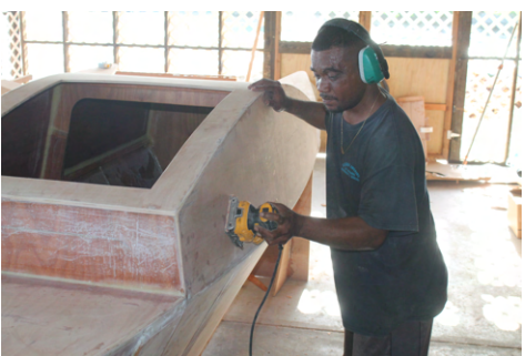
(c) The entire deck and cabin surface is sanded in preparation for glassing.
