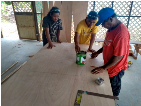
(c) A tin can is used to draw the radius of the internal cut-out.
