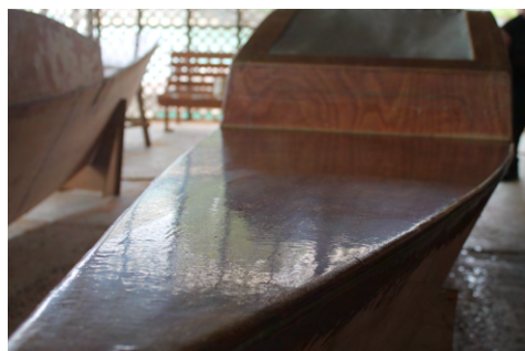
(a) One hour after glassing another layer is applied wet-in-wet (a 'flow-coat') to reinforce the rot-resistant epoxy layer.
