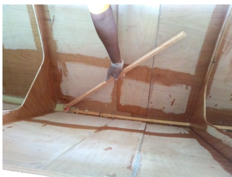
(c) Application of the keel fillet
