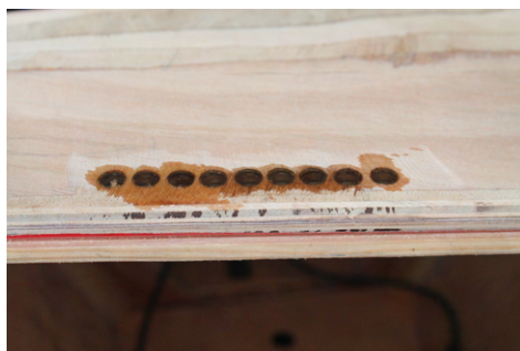
(c) The holes are filled with epoxy resin. The plywood will absorb the resin, so the holes will need a couple of refills.
