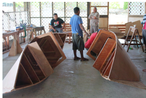
(d) Both hulls are treated in parallel with three layers wet in wet. To ensure the job is finished in time, some preparation and planning, and organization of the crew is required.
