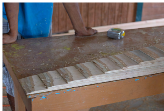
(b) The scarf bevels depicted are halfway through being planed. Every line of the steps should be parallel for a good result.
