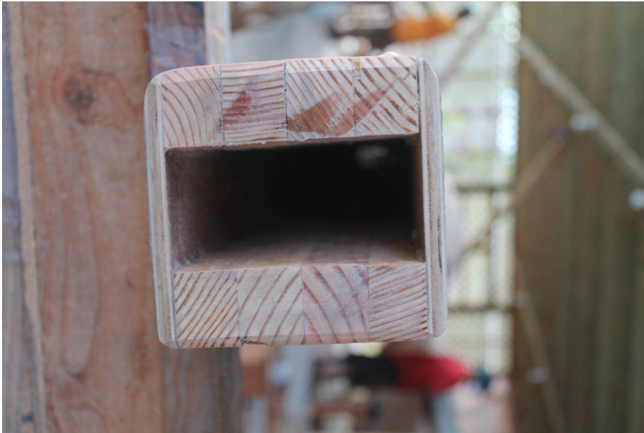
Figure 35: The rectangular and hollow cross section of the beams. The lumber is positioned on the top and bottom to take the bending loads while the vertical plywood works as a shear web.
