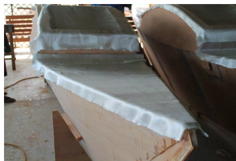
(b) The glass fiber is cut to the size of the hull with an overlap of three fingers to reinforce the edges.
