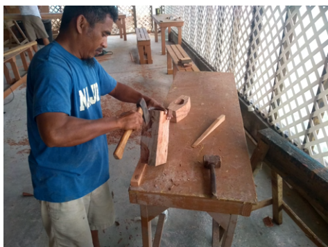
(a) The mast bases are carved from large pieces of local hardwood.
