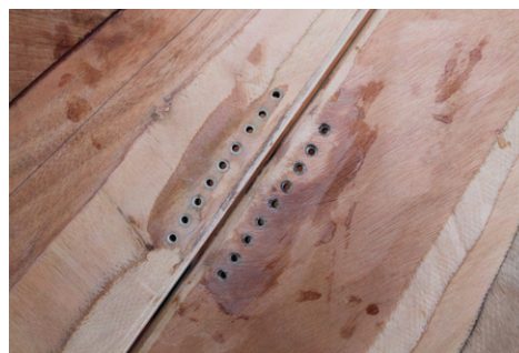
(d) After the resin in the holes has cured they are re-drilled carefully (without cutting into the wood) to the required diameter.
