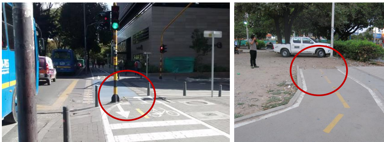
Figure 6: Bad practice examples of current cycling infrastructure
